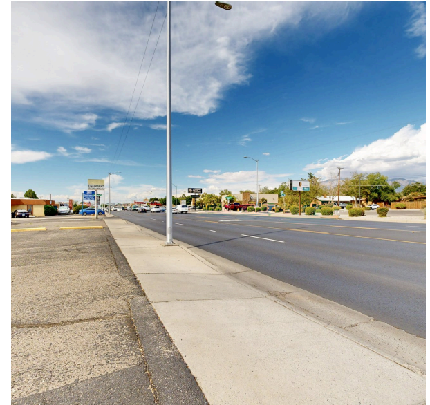
San Mateo Blvd looking south — six lanes, up to 47,209 VPD
