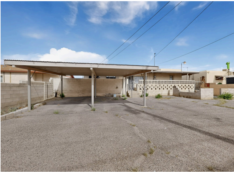
Rear yard — steel carport with covered parking, CMU walls
