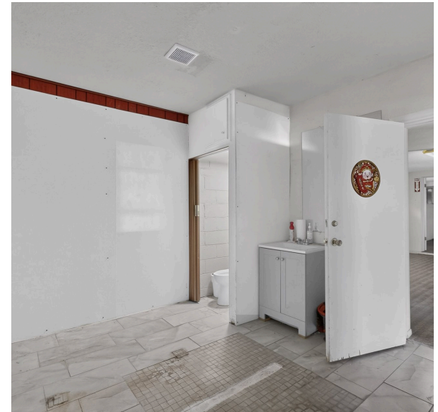
Laundry / utility area with W-D connection
