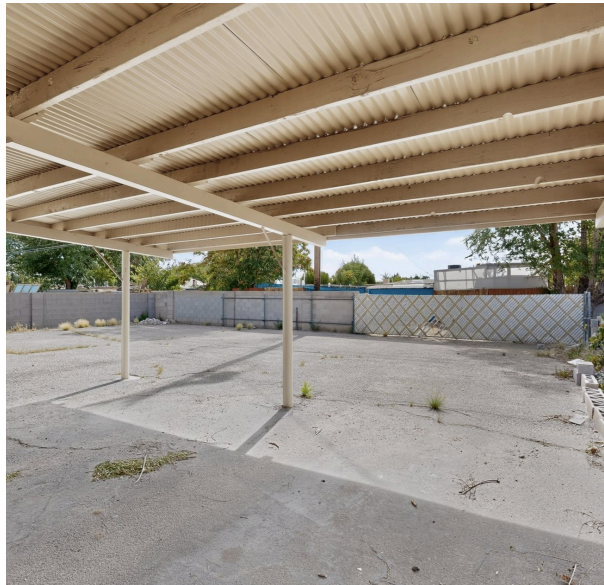
Under the rear carport — covered parking
