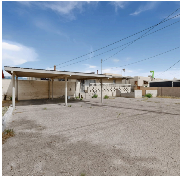
Rear yard toward the alley
