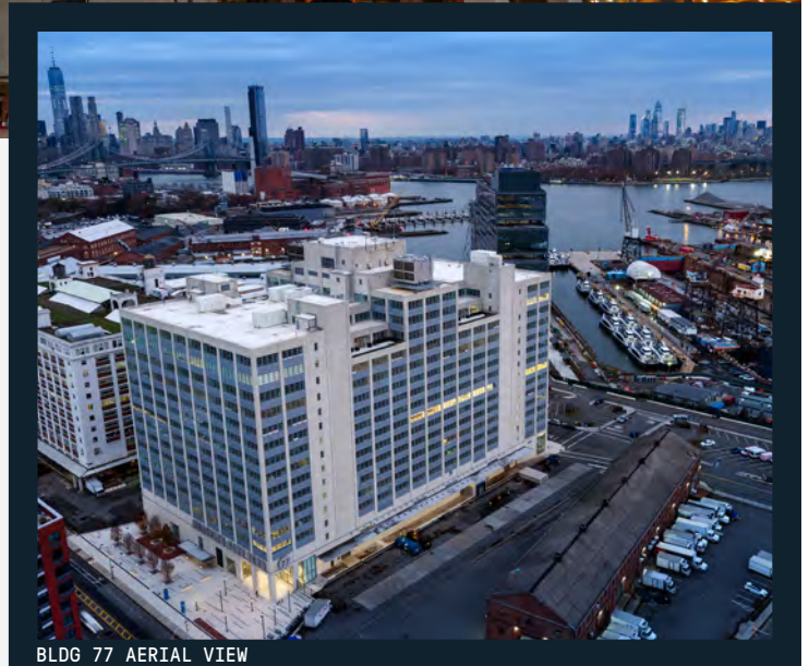
BLDG 77 AERIAL VIEW
