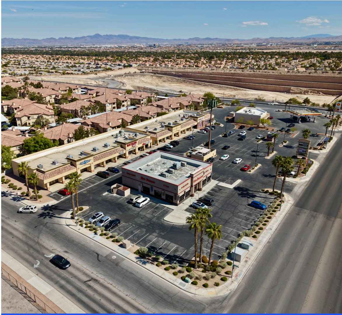
High-Visibility Retail Space Along the Durango Drive Corridor
