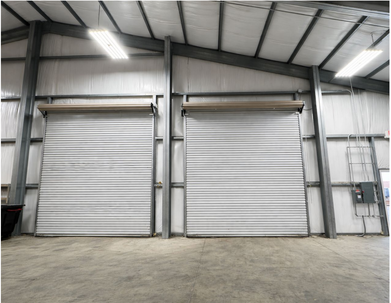
Secondary Building (10,000 SF)
