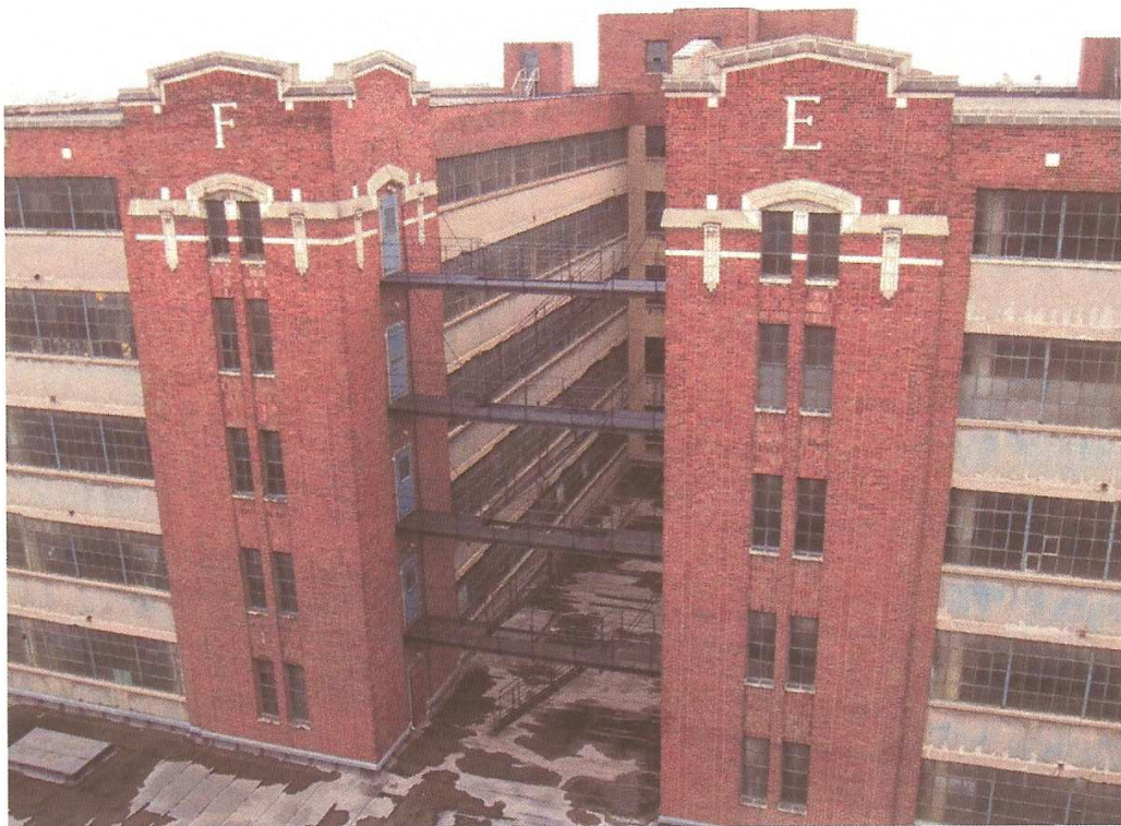
Buildings E and F north side.
