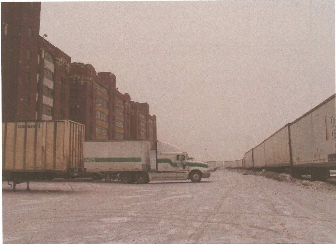
Rear (south) side of Buildings D, E and F.
