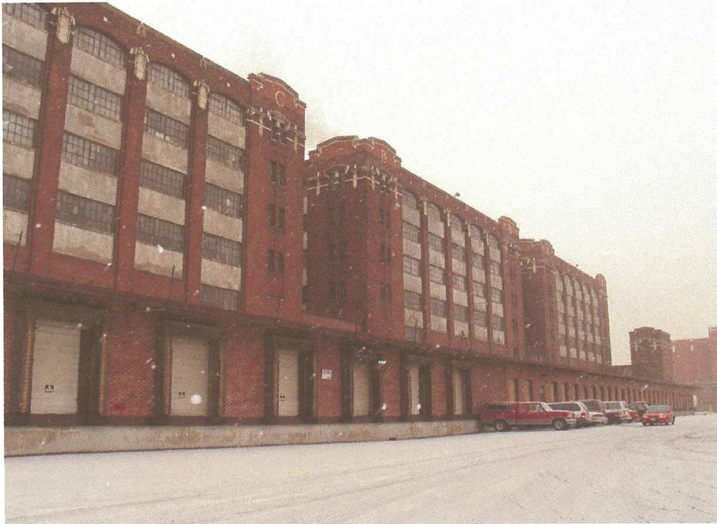
Buildings A, B and C north side from parking area.
