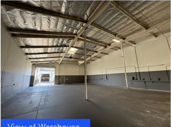
View of Warehouse
