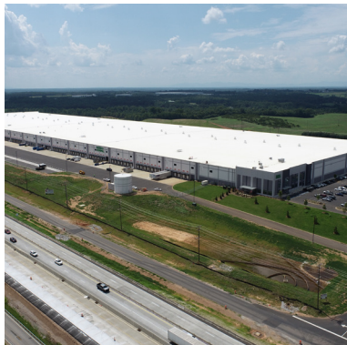
DHL/Mann+Hummel \pm 1.4 -MSF distribution facility spec-to-suit
