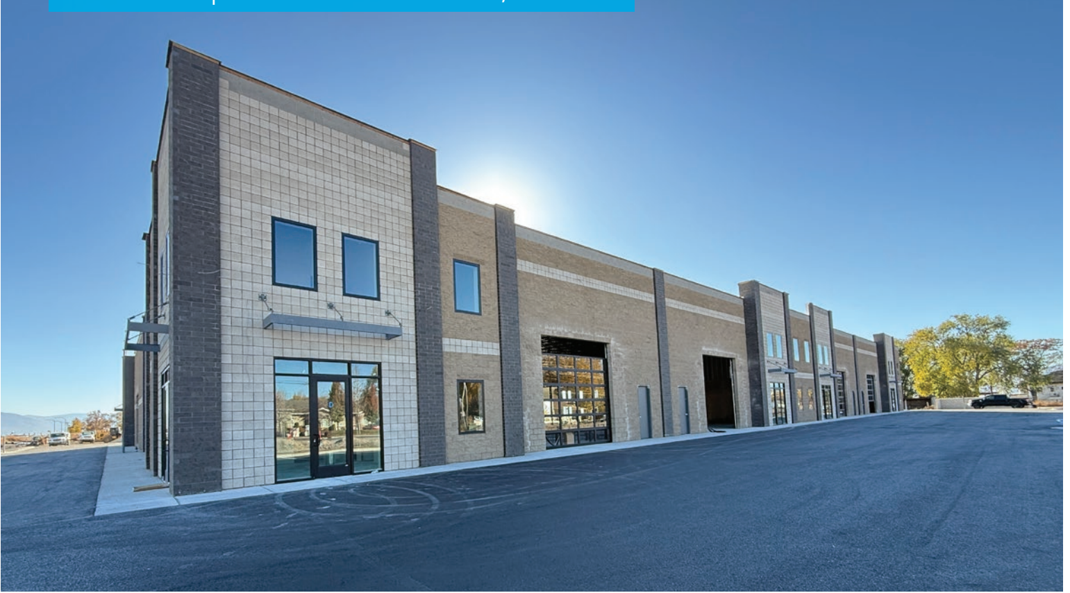
Photos | 3155 W Center Provo, Utah
