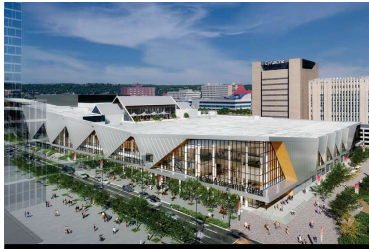
Convention Center Renovation Full Office Renovation
