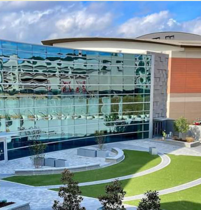
GAS SOUTH CONVENTION CENTER
