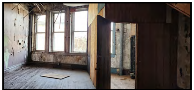
2nd Floor Cotton Avenue View
