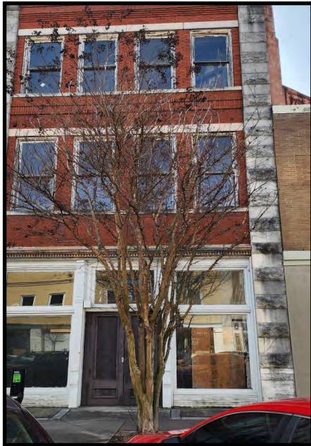
1st Floor Cotton Avenue Entrance
