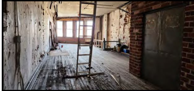
3rd Floor Cotton Ave View/Brick Elevator Shaft
