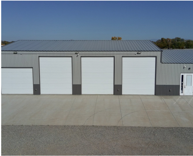
South elevation — four overhead doors and man door, concrete apron
