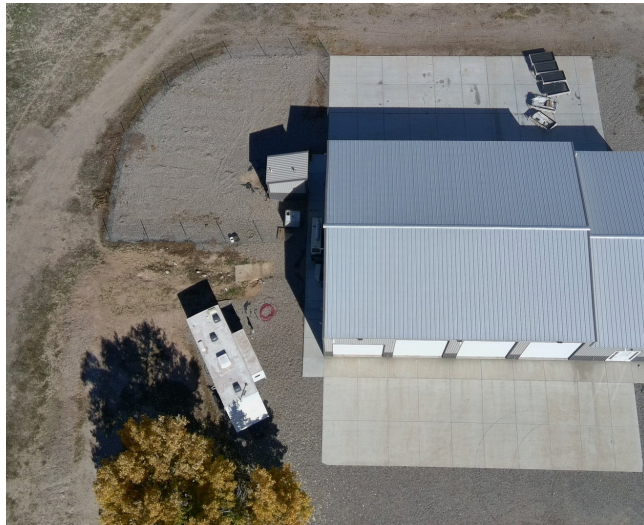
Nadir — roof, aprons north and south, RV hookup
