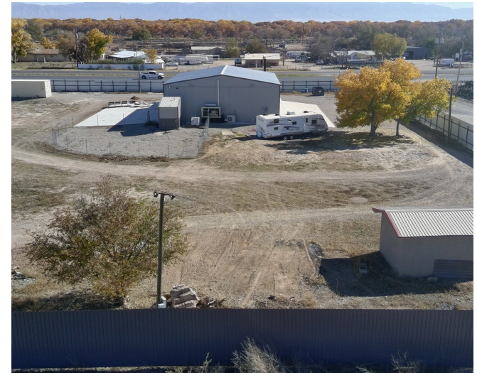
Looking east — north pad, storage shed, loop drive
