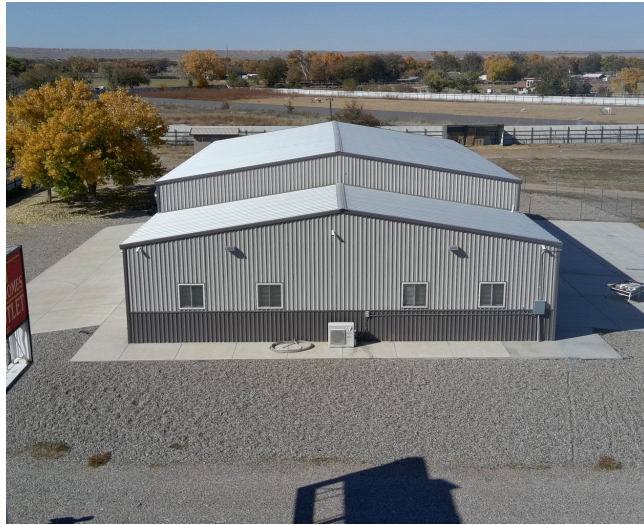
East gable — two-level core with windows; north pad at right
