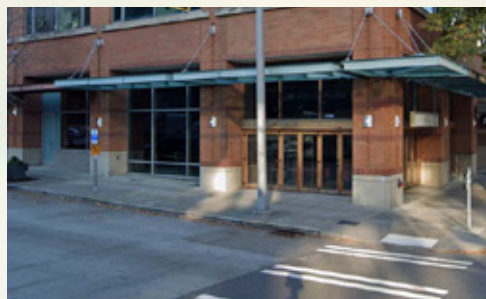
Elevation view from Thomas St
