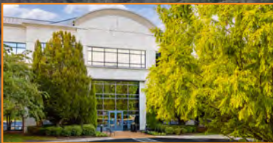
PETER JEFFERSON PLACE VII 652 Peter Jefferson Pkwy
