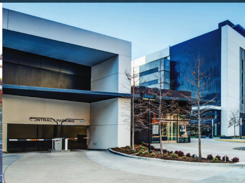
VALET & VISTOR PARKING GARAGE
