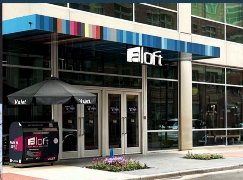
ALOFT HOTEL LOCATED IN ONE CITY PLACE
