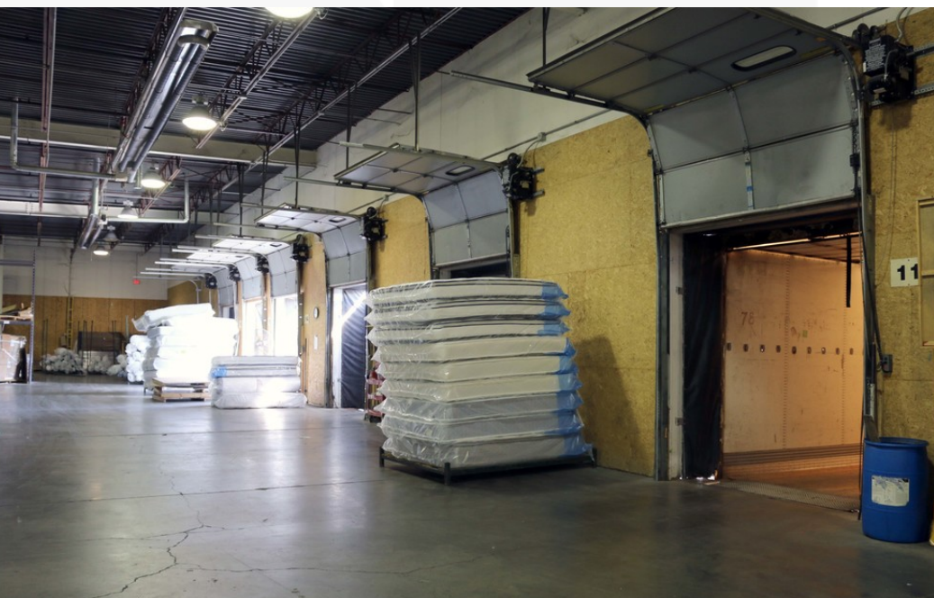
15 interior dock-high doors on east side
