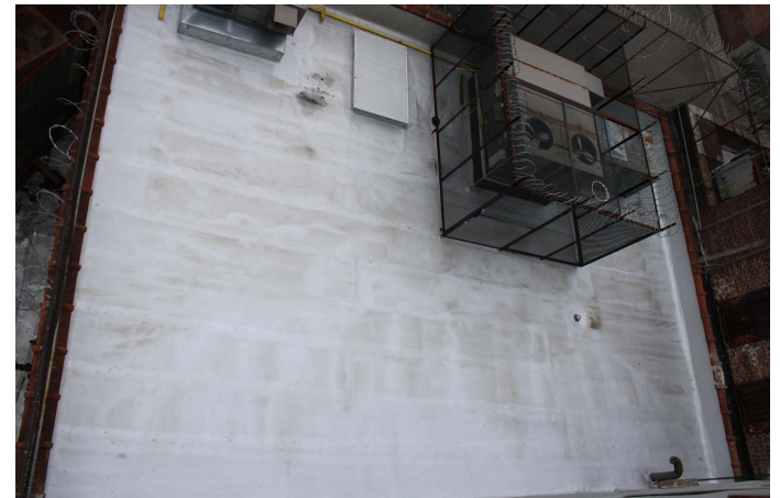
Adjacent Roof Access
