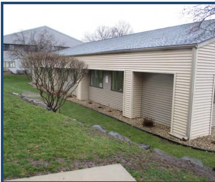
West Elevation of Building Facing East
