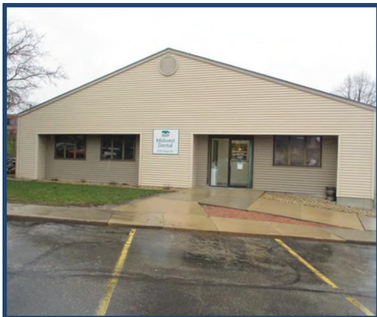
South Elevation of Building Facing North
