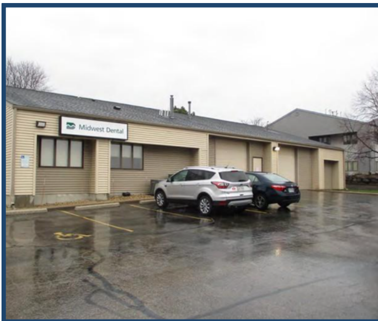
East Elevation of Building Facing West
