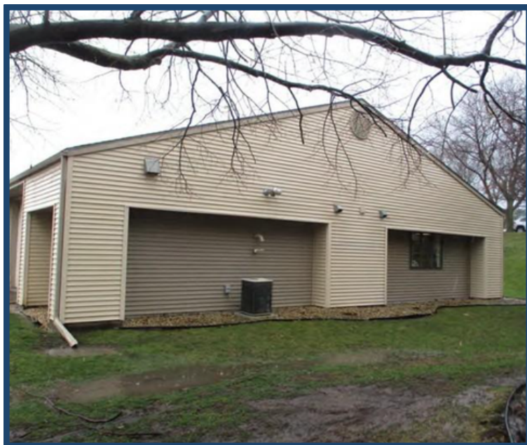
North Elevation of Building Facing South
