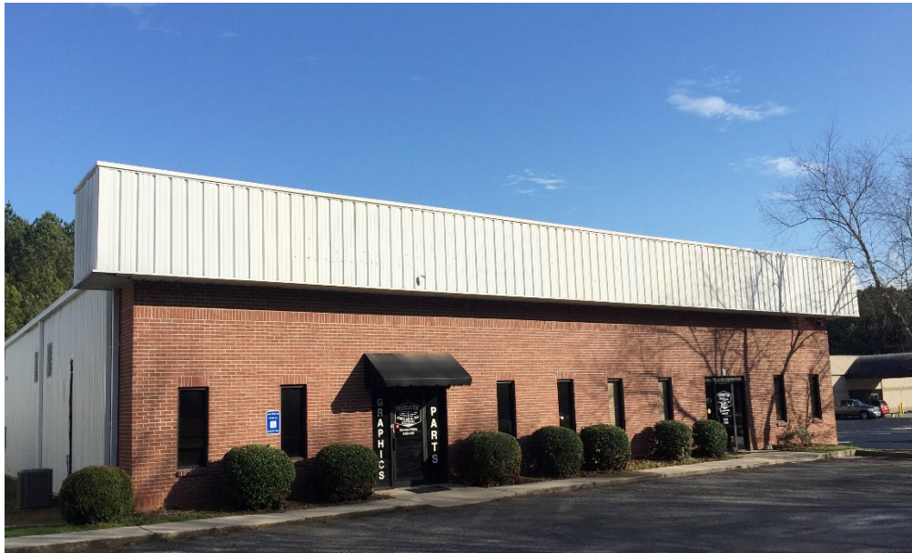
Property Profile- Building 116
