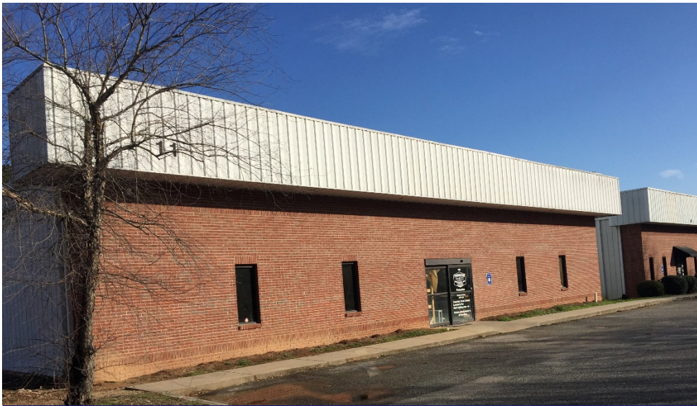
Property Profile- Building 110
