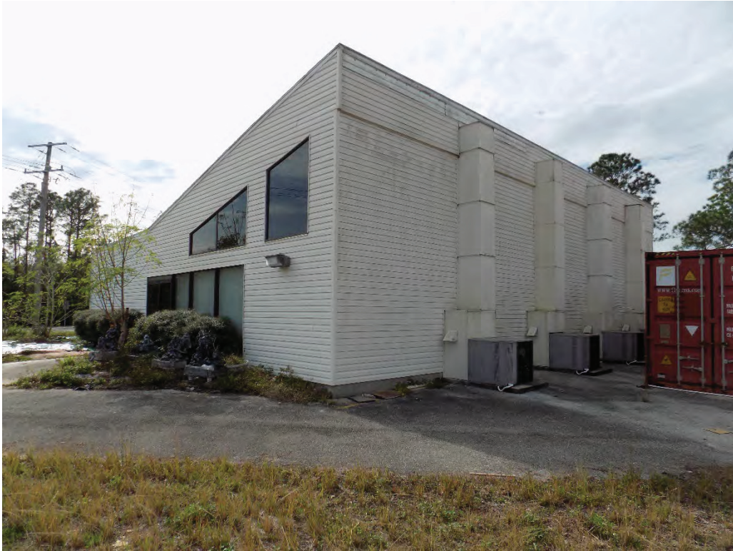
NE corner of subject building looking SW
