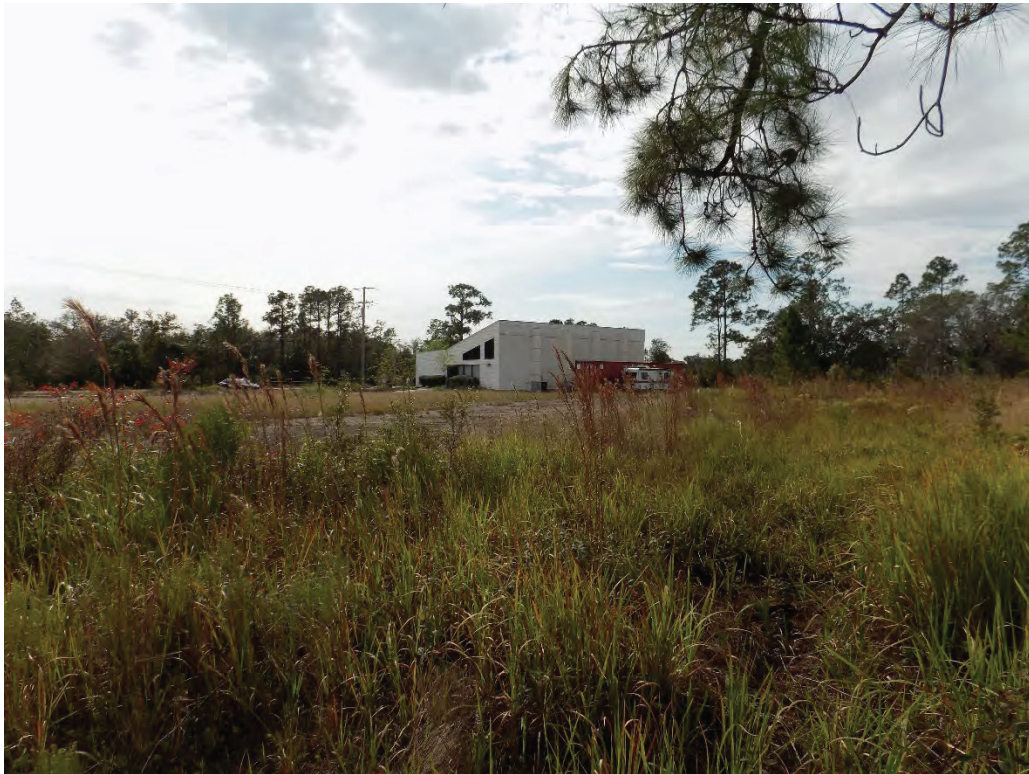
Looking SW from the NE corner of subject property
