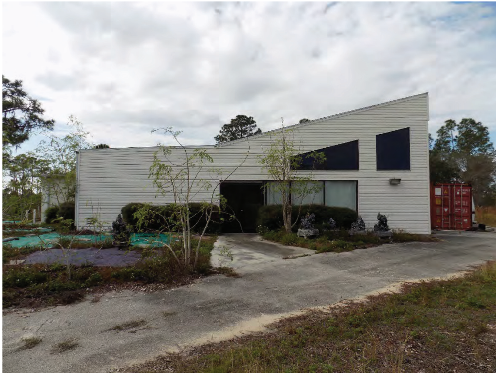
Main entrance of subject building looking NW from SE
