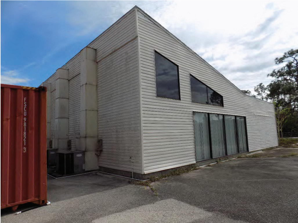
NW corner of subject building looking SE
