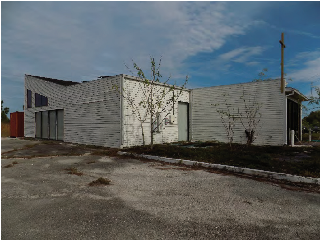
SW corner of subject building looking NE
