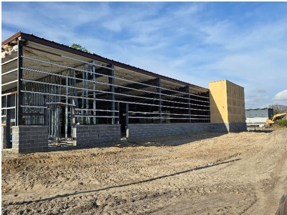
Typical View of Subject Exterior
