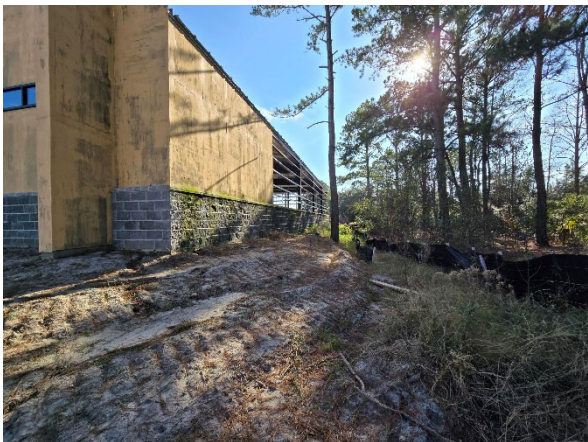
Typical View of Subject Exterior
