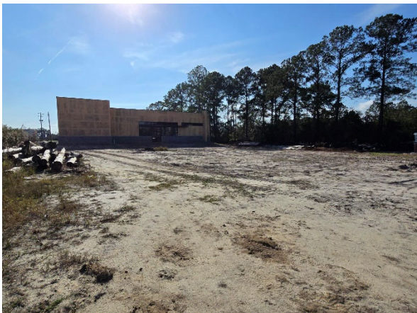
Typical View of Subject Exterior
