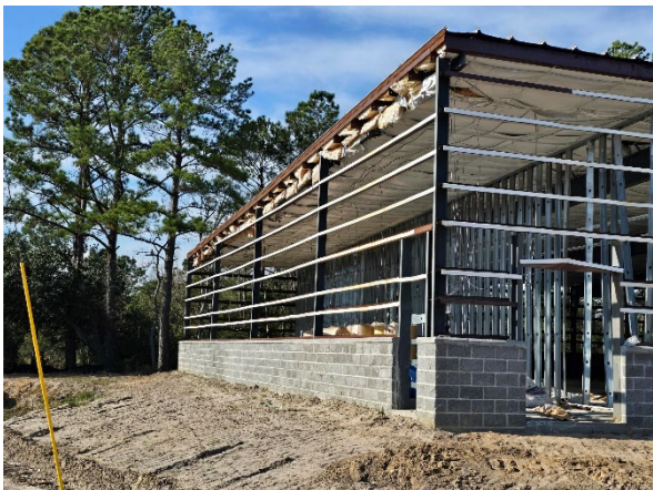
Typical View of Subject Exterior
