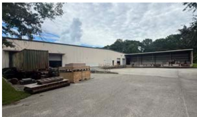
Loading Docks & Covered Loading Platform
