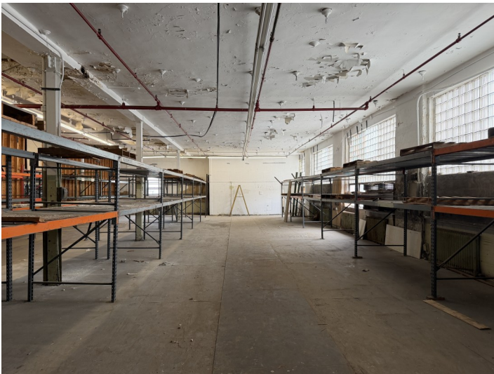
Second Floor Warehouse
