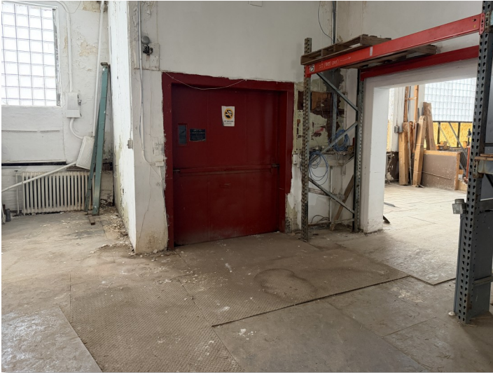
Second Floor Warehouse
