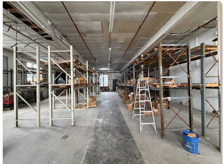
Second Floor Warehouse
