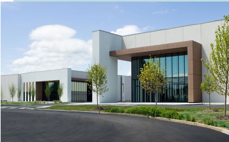
Affinius Capital and Trammell Crow Co. brought online Springbrooke Trade Center, a spec project totaling 484,000 square feet in an infill area of suburban Philadelphia. The project, which wrapped up in 2021, is now fully leased. Photo courtesy of Affinius Capital
